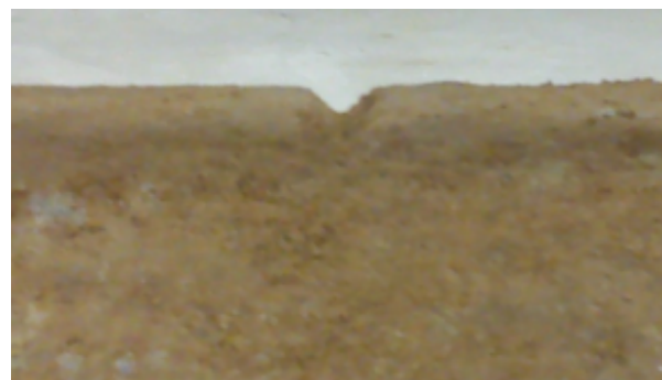
Figure 8: Photo of the pilot channel of the second embankment.
