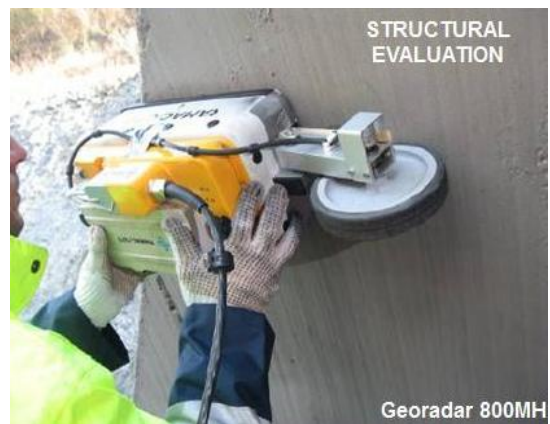
Figure 4- Tunnel structural evaluation [6]
