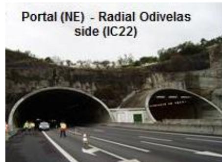
Figure 1- View of the tunnel portals
