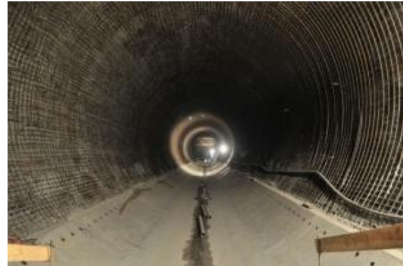
Figure 3 – Concrete casting in site (bottom) (EDP, 2011)
