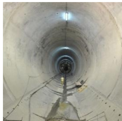
Figure 1 – Reinforced concrete liner (interior view) (EDP, 2011)
