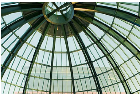
Fig. 4.3.2.8. C.C. Colombo – detalhe cúpula central
