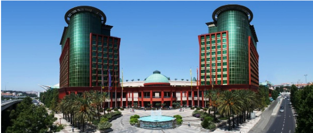
Fig. 4.3.2.1. Centro Comercial Colombo – Fachada Principal
