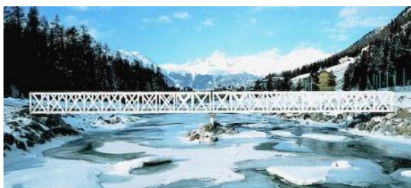
Figura 2.17. Ponte pedonal Pontresina [2.10]
