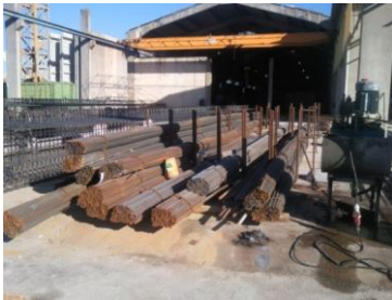
Figure 2.1 – Proper storage of reinforcement rebars.
