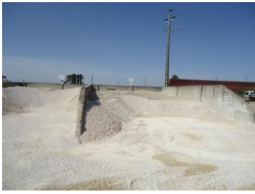
Figure 2.2 – Proper storage of different aggregated in gravel bails.
