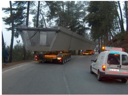
Figure 2.5 – Truck transporting a precast beam (Solonha, 2005).
