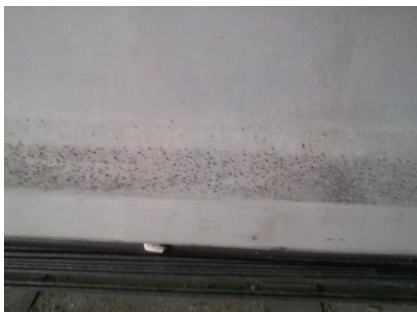
Figure. 3.3 – Piece before application of the aesthetic treatment (honeycombed).
