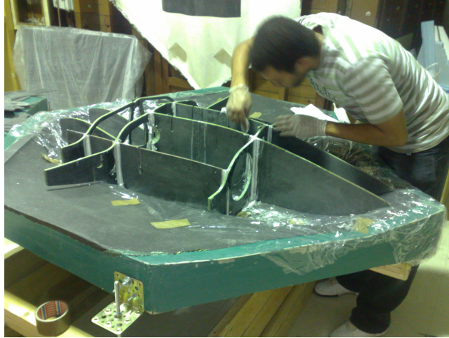
Figure 4.24: Application of the epoxy resin.
