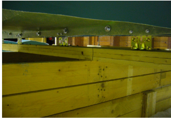
Figure 3.10: Halves of the moulds bolted.
