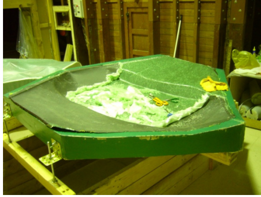
Figure 4.4: Removing the peel ply, the net and the resin excess.
