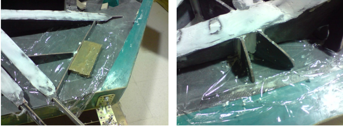
Figure 4.36: Gluing non-structural pieces.
