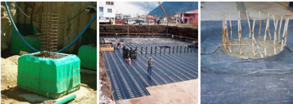
Figure 1 - Types of foundations that can be protected with waterproofing: isolated foundation footings, mat-slab foundations and pile heads [3] [w<sub>1</sub>][w<sub>2</sub>]
