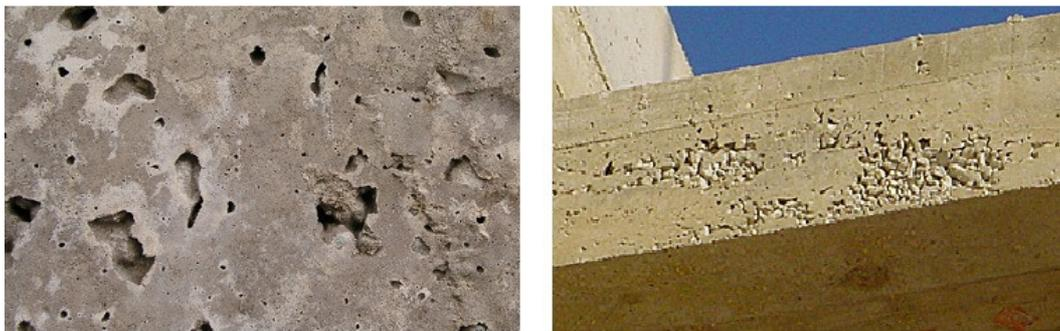
**Figure 13** - Anomalies during execution: voids and segregation of concrete [w<sub>4</sub>][w<sub>5</sub>]
