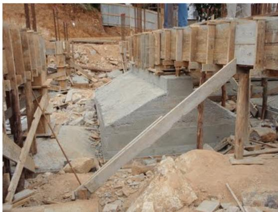
Figura 2.6 - Sapata corrida [w<sub>7</sub>]
