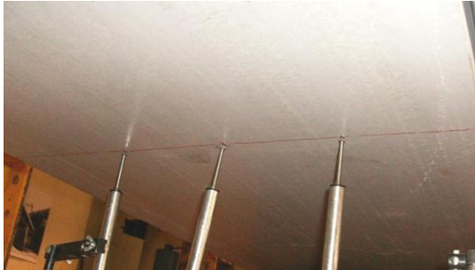
Figure 10 – Instrumentation for the service characterization test.
