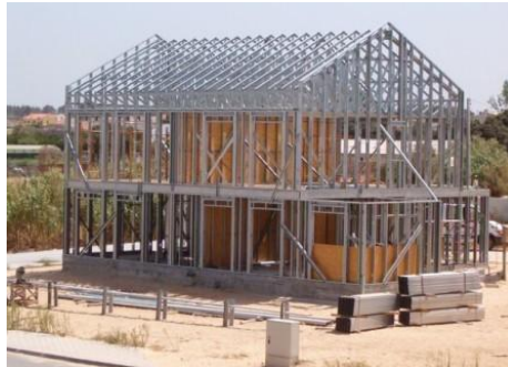
Figure 3 – Light Steel Frame (Engenharia Civil Wordpress, 2011)
