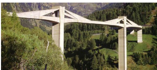
Figure 2 – Ganter Bridge, Switzerland [4].
