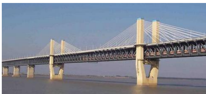
Figura 1.12 – Ponte Wuhu, China [1.11].
