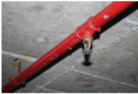
Image 2.5 - Sprinkler and supplying system
