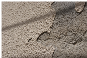
Figure 5 – Example of a “textured” paint surface texture.
