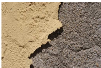
Figure 6 – Example of a “smooth – plastic” surface texture.
