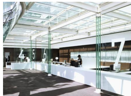
Figure 2 - Glass columns in a convention center in Saint-Germain, France [2].
