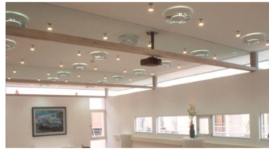
Figure 4 – Use of glass-wood composite beams in a conference room [4].
