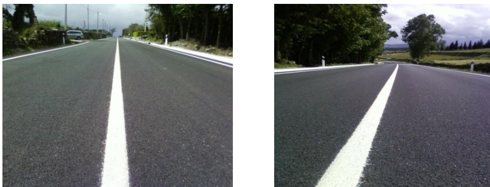
Figure 6.1 – Pavement of EN 226 after rehabilitation
