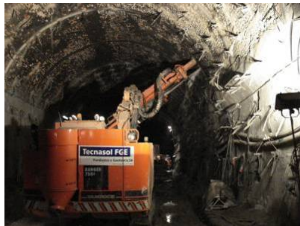
Figure 6 – Soil nails execution
