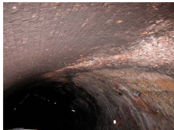
Figure 3 – Vault deformation [2]
