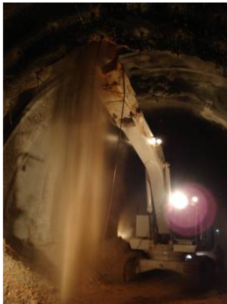
Figure 8 – Excavation with cutter-loader
