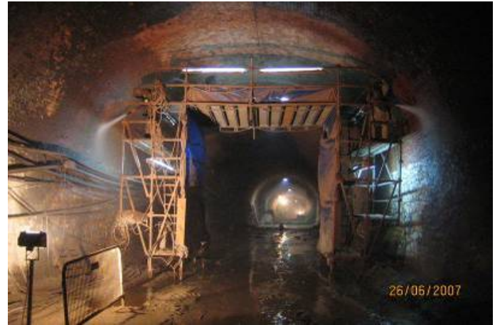
Figure 11 – Masonry cleaning by wet shooting a mix
