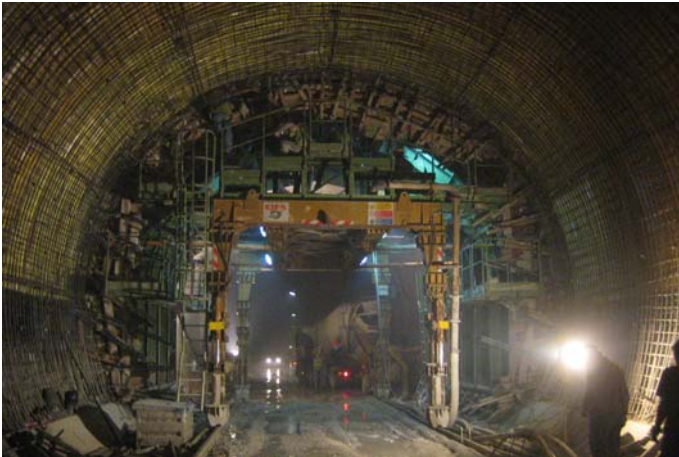
Figure 10 – Metallic Formwork
