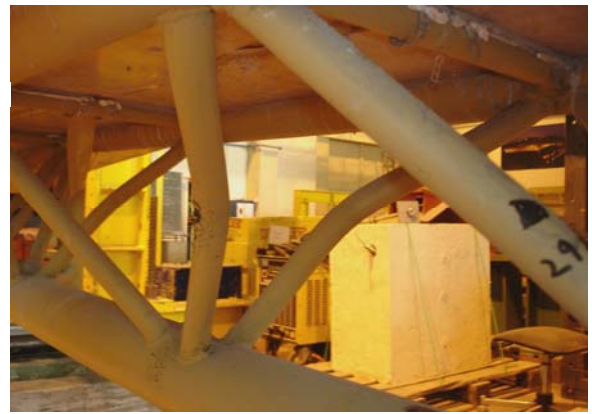
Fig. 15 -Buckling of compressed diagonals.
