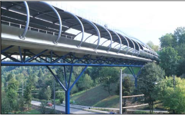
Fig. 2 - The Nesenbachtal Bridge, Germany.
