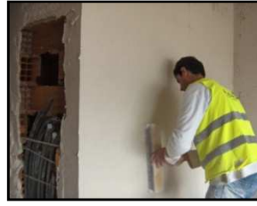
Figure 3: Straightening with a spatula
