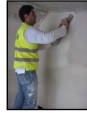
Figure 4: Application of a finishing coat with trowel
