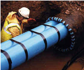
Figure 3.8 - Sublining technique, during application (Subterra, 2003)
