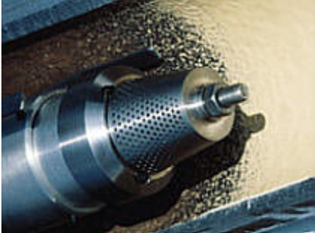
Figure 3.3 – Spray Relining Technique: detail of the spray cannon (Subterra, 2003)
