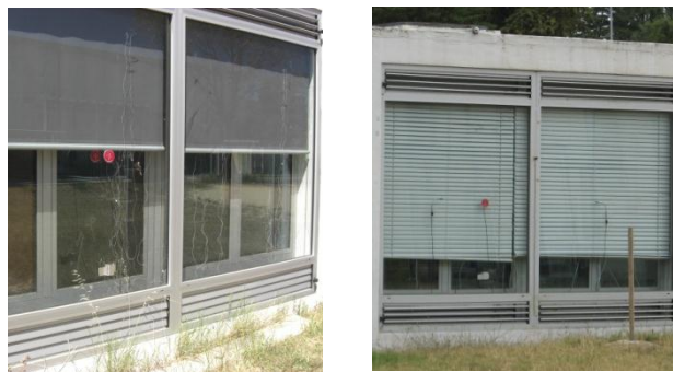
Test cell experiments of double skin façade with roller and venetian blinds.
