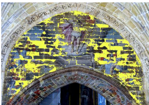
Result of a Maximum Likelihood Classification for the lacunae in a wall painting
