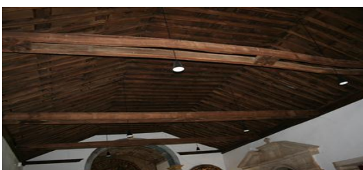
Roof, Church of São Vicente de Castelo Mendo, XVI Century,
