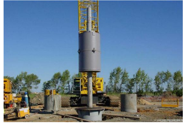
Dynamic load test on experimental pile (800 mm) with a 20 ton hammer
