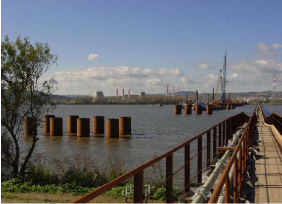
Foundation piles of a bridge
