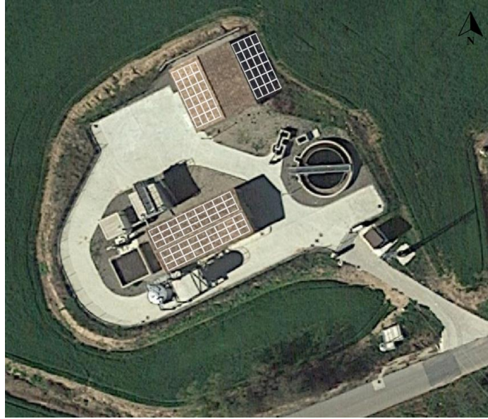
Figure 19: PV panel distribution on the sewage treatment plant roof.
