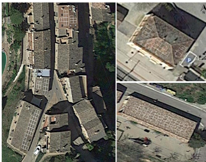
Figure 17: PV panel distribution on the municipal building roofs.
