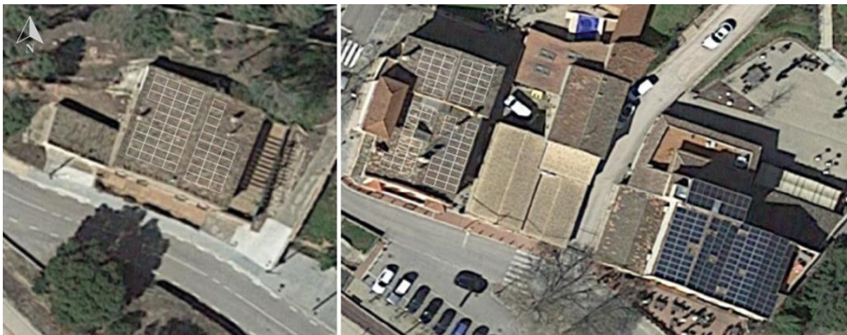
Figure 23: PV panel distribution for the restaurants.
