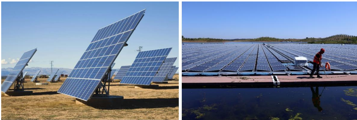
Figure 4: Solar farm with a module tracker system (left) 20 and Europe's largest floating solar park located in Portugal (right) 21 .
