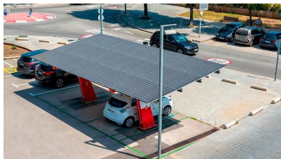
Figure 25: Example of a solar-powered electric vehicle charging station 91 .
