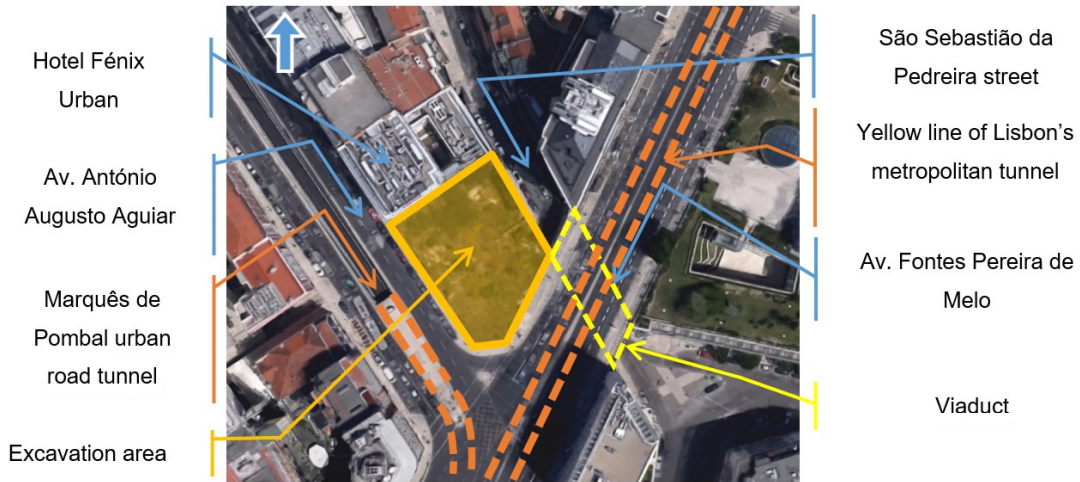
Figure 1: Aerial view of the construction site (Source: Google Earth)
