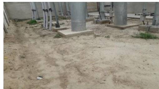
Figure 16: Boundary wall support soil rectified
