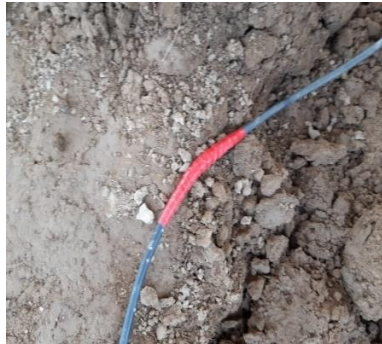
Figure 14: Cable repair with HT & PVC tape
