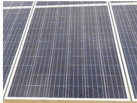
Figure 19: Damaged module replaced with a new module
