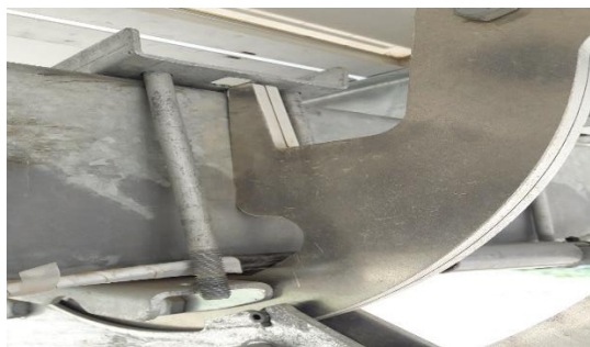
Figure 20: New pile head installed at a tracker
