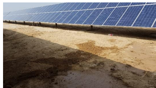
Figure 12: Cable trench slip rectified after pumping out water
