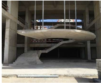
Figure 4 - Structure of the staircase.
