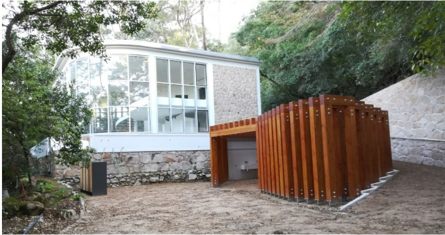
Figure 9 – Building after rehabilitation
