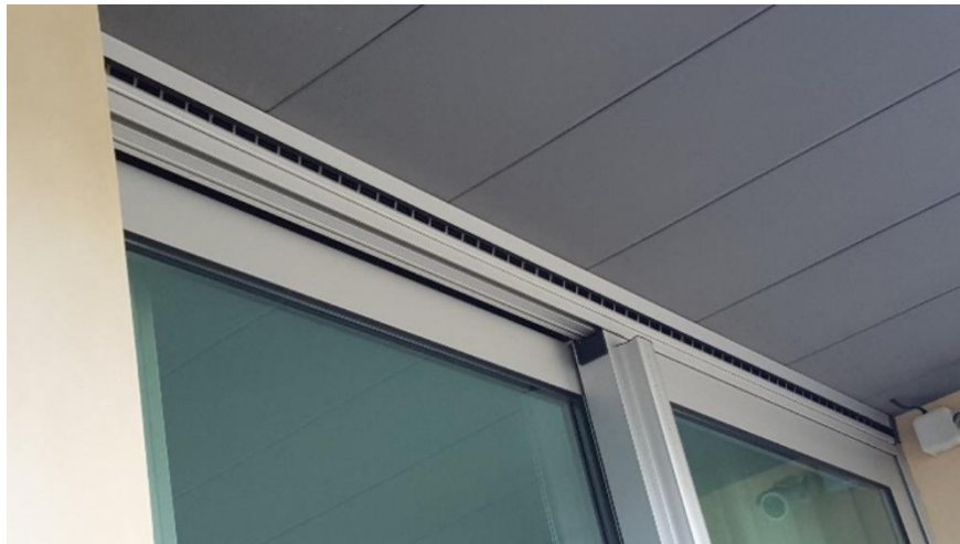
Figure 12. Example of air intake openings on living-room window
