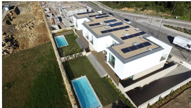
Figure 19. Overview of townhouse rooftop and RES installed (Image obtained from Belas Clube de Campo)
