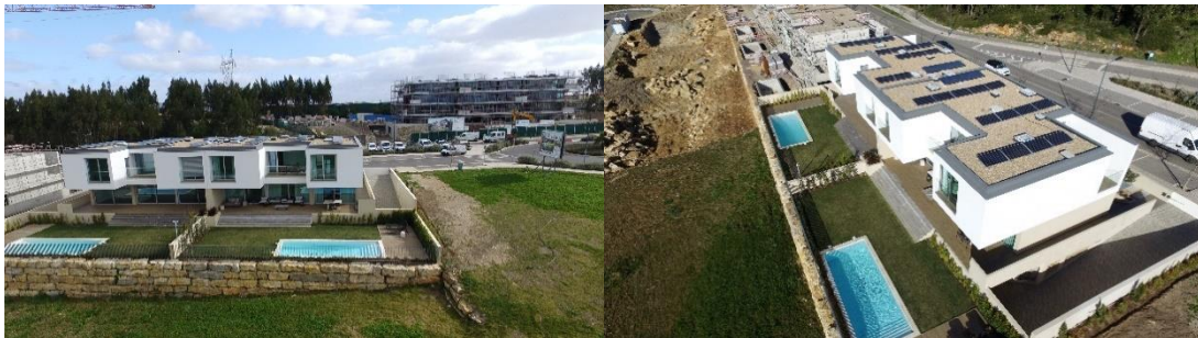
Figure 7. Back view and top view of Townhouse 307 (Images obtained from Belas Clube de Campo)
