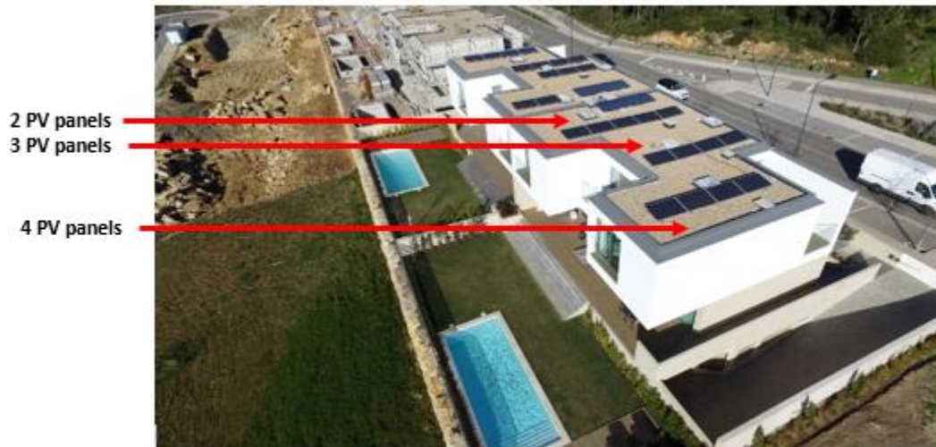
Figure 21. Proposed installation of collector and PV panels
