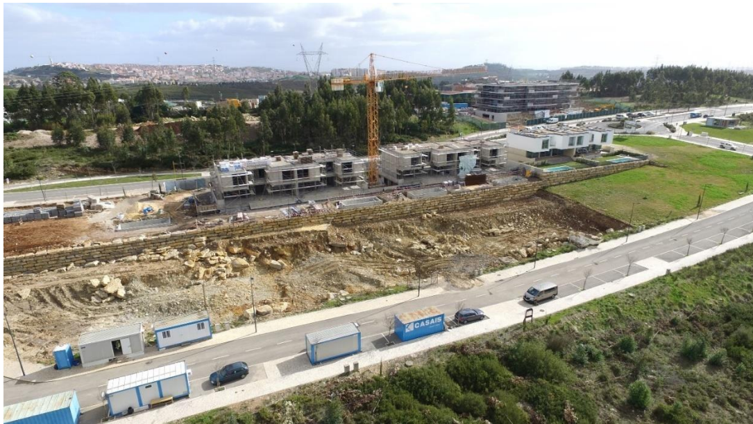
Figure 5. Current status of stage 3 (Image obtained from Belas Clube de Campo)
