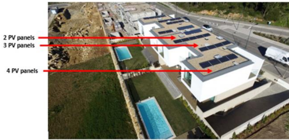
Figure 6. Proposed installation of PV panels
