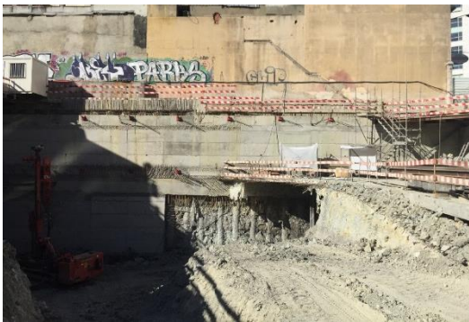
Figure 16: Slab bands at 17/08/2016.
