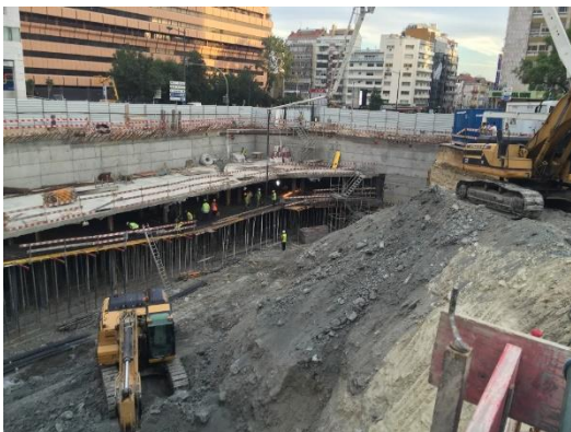
Figure 17: Slab bands at 20/09/2016.
