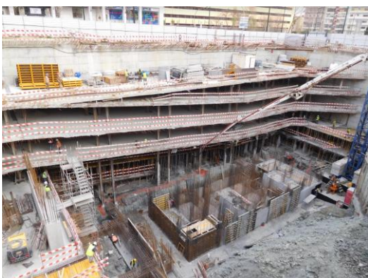
Figure 18: Slab bands at 23/02/2017.
