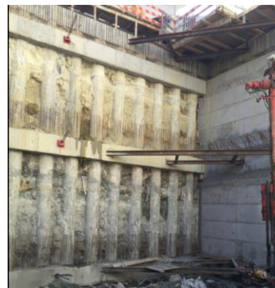
Figure 1: Steel Corner Shoring [FPM41].
