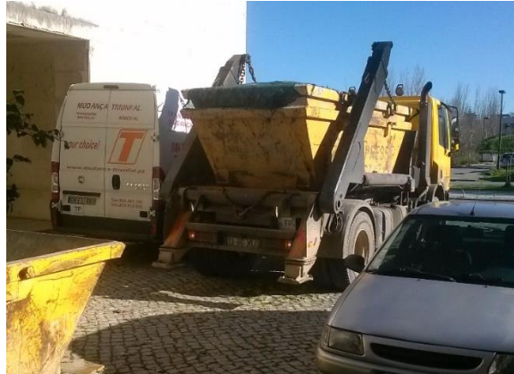
Figure 6 Construction waste transport
