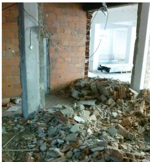
Figure 5 Demolitions in the project
