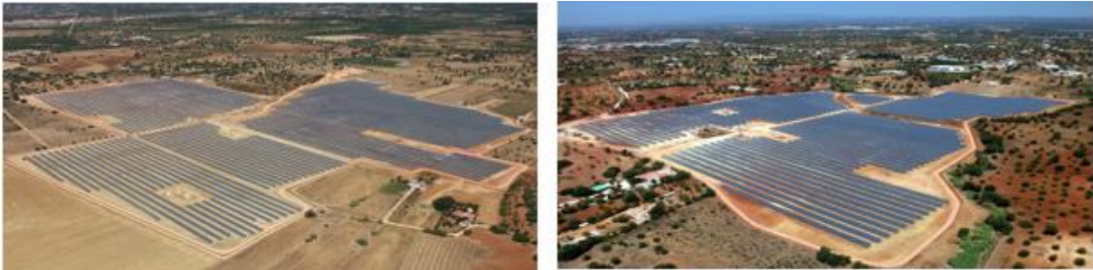
Figure 42 Avalades, Silves PV plant (left) and Ferreiras, Albufeira PV plant (right) [80].
