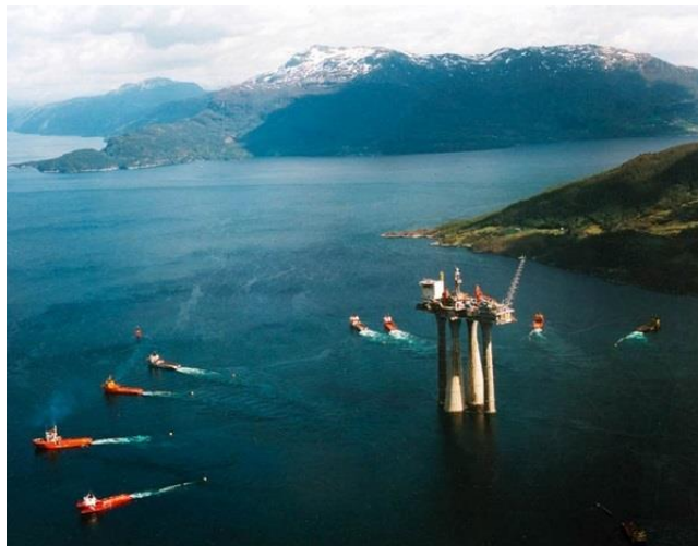
Figure 6: Troll A offshore platform, built in land and moved across the water, in North Sea [3].
