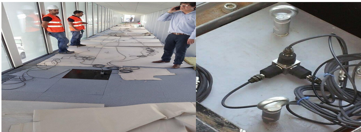
Figure 5.5-Ambient vibration records after completion of the footbridge
