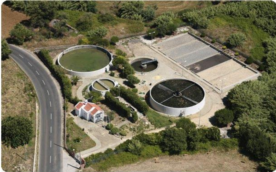
Figure 2 - Póvoa da Galega's Wastewater Treatment Plant (SimTejo, 2009)
