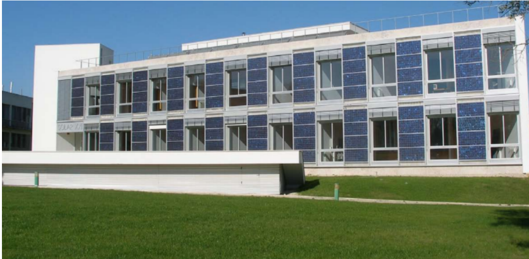
Figure 2.1: LNEG Solar XXI building after renovations, South facade [9].
