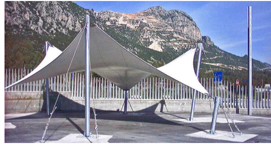
Membrane - tension stresses
