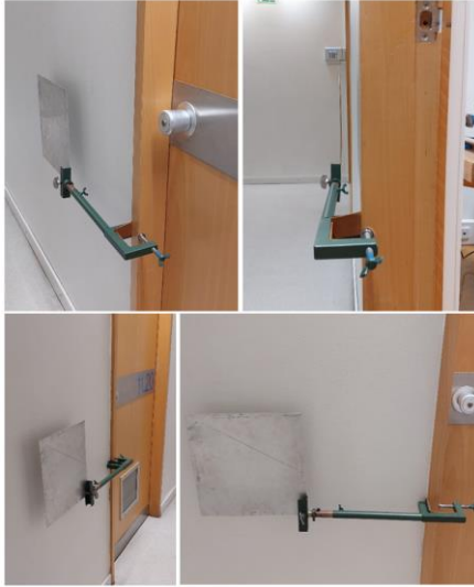
Fig. 21 - Installing the metal plate (target) behind the wall
