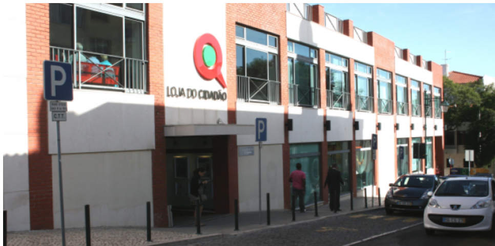
Figure 2.1: Cascais Center photo [14]
