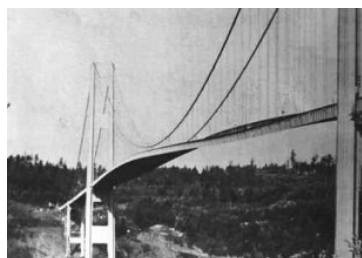
Figure 2.5: Flutter catastrophic phenomenon in Tacoma Narrows bridge, Washington USA
