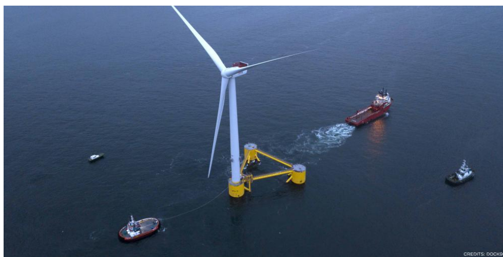
Figure 2.4: WindFloat Atlantic off the coast of Viana do Castelo, Portugal. Source: Dock90
