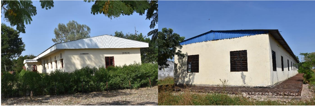
Figure 3.5. VC Building (left) and the Lecturers' Building (right).
