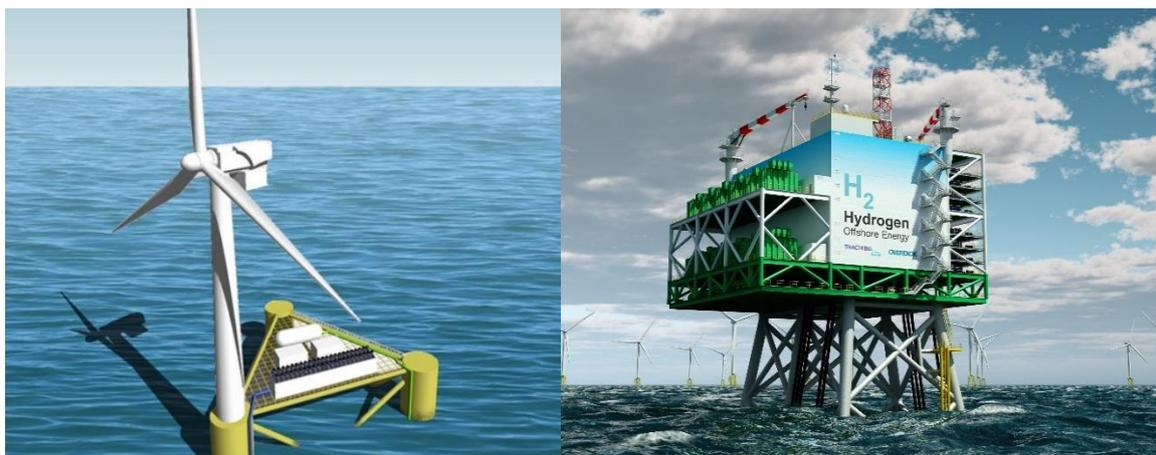
Figure 26 Decentralised production, from Dolphyn project [60] and centralised production, from Tractebel [61]
