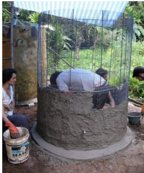
Figure 12: Ferrocement water tank [36]
