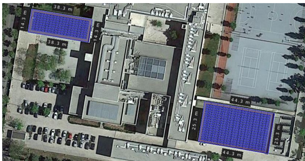
Figure 4.5: PV system display on buildings E (left) and G (right).
