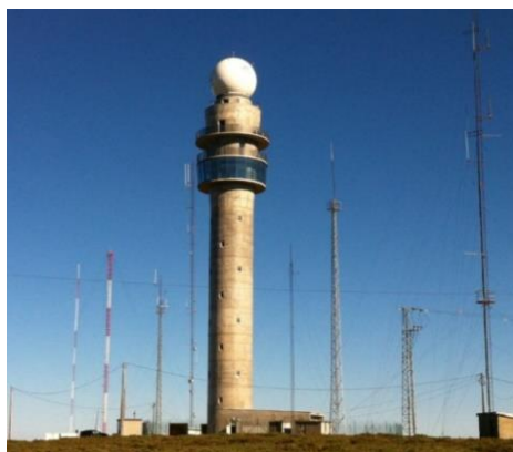
Figure 3.15-Weather radar of Arouca. Photo taken by: Sérgio Barbosa.
