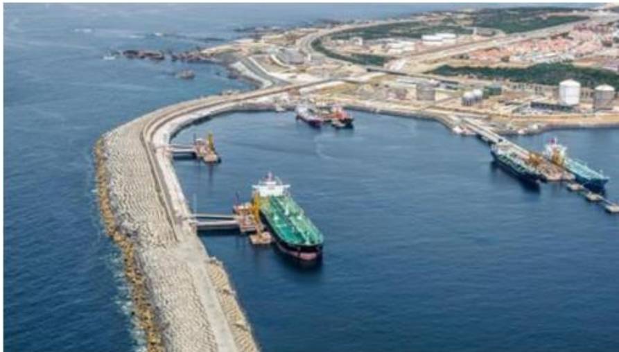
Figure 3: Liquid Bulk Terminal of Sines
