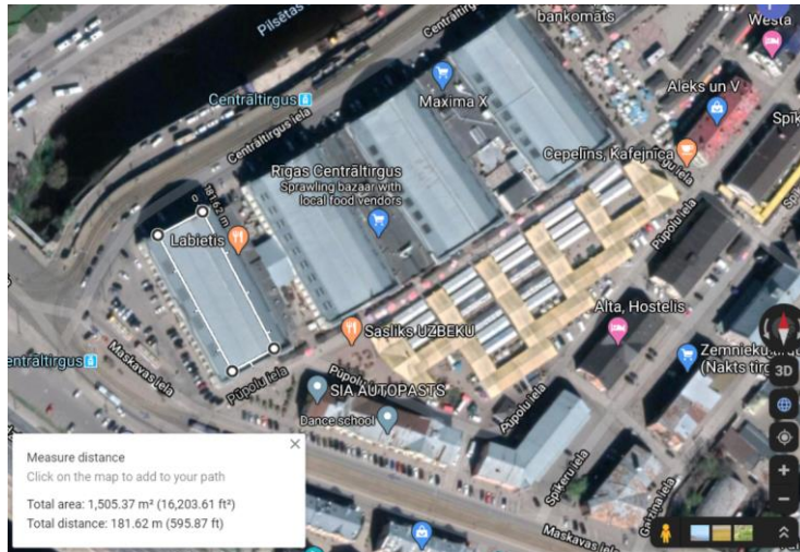
Figure 43: Example PV system on the roof of one of the four Riga main station halls [101].
