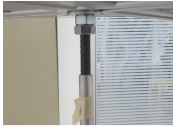
(b) Screwing fixation.
